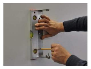
2) Drill the holes using screws and dowels that can support the weight of the MIDIReel according to the type of bracket used.
